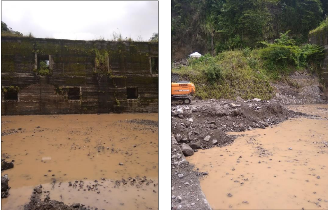
Figure3. Check dam excavation activity
