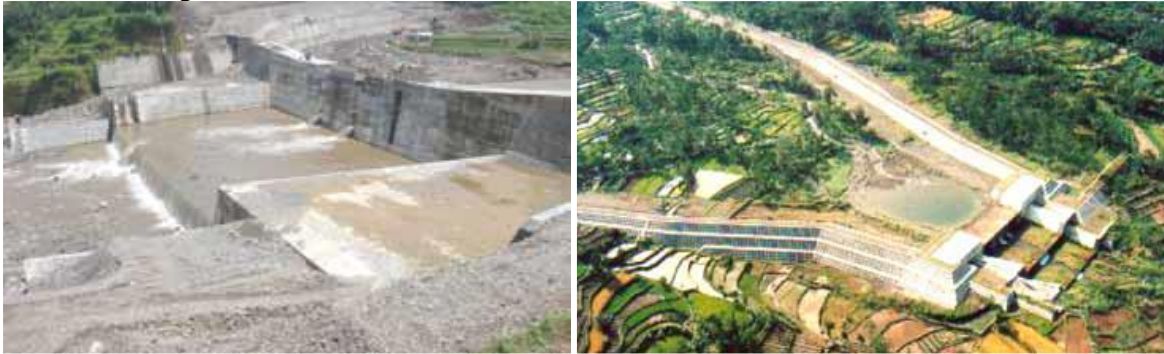
Figure 2. A check dam (left), and lava pocket (right) in Batang River, Magelang
