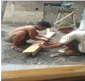
Gambar 9 : set and close the formwork
