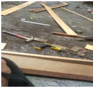
Gambar 8 : make size on formwork material
