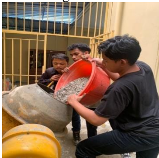
Gambar 10 : liquid concrete manufacture
